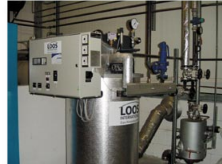
Our steam boiler with a pressure of 100 lbs is used to test each piece of equipment before delivery
